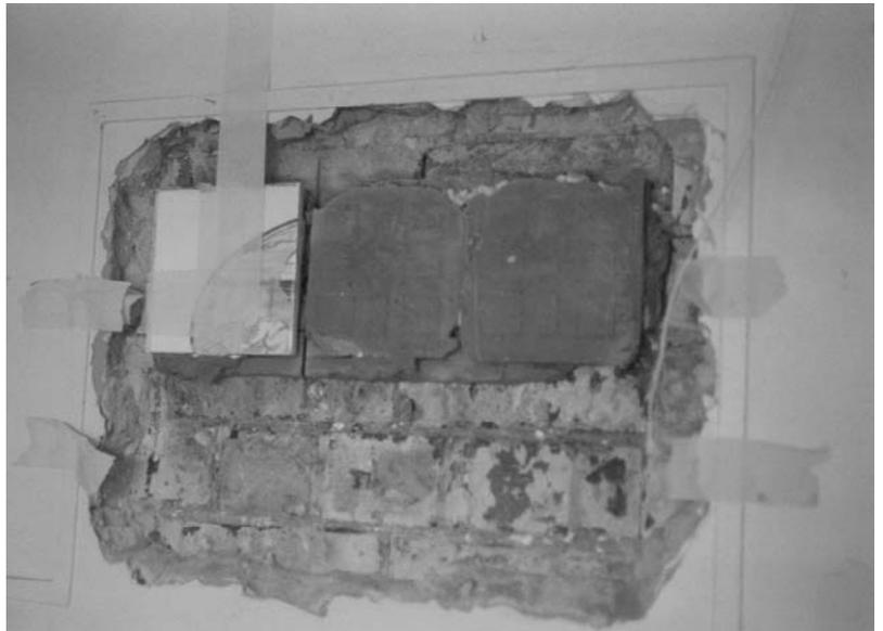
always release the tile, along with its adhesive layer still attached, from the substrate (Figures 5.34–5.36).
