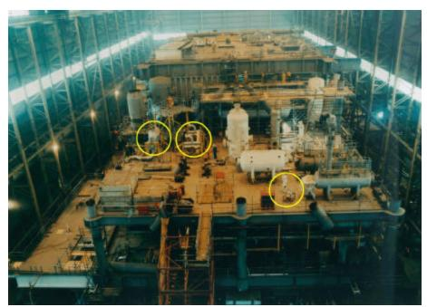
Figure 2.4.6 – Compression Cooling Printed Circuit Heat Exchangers Installed on a Gas Platform (Courtesy of Heatric Ltd)
