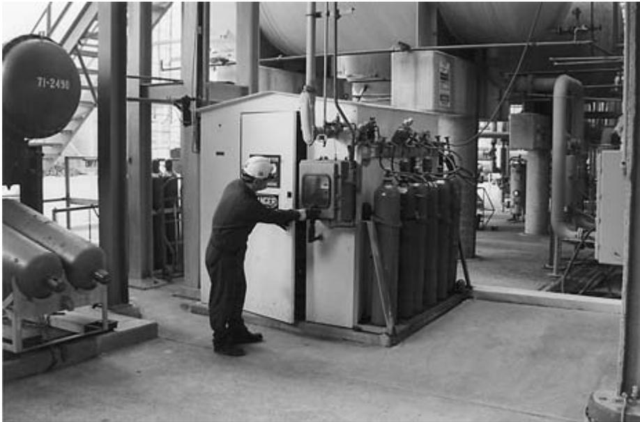
FIGURE 2–23 Typical pressurized and purged analyzer buildings found in chemical plants handling flammables.
