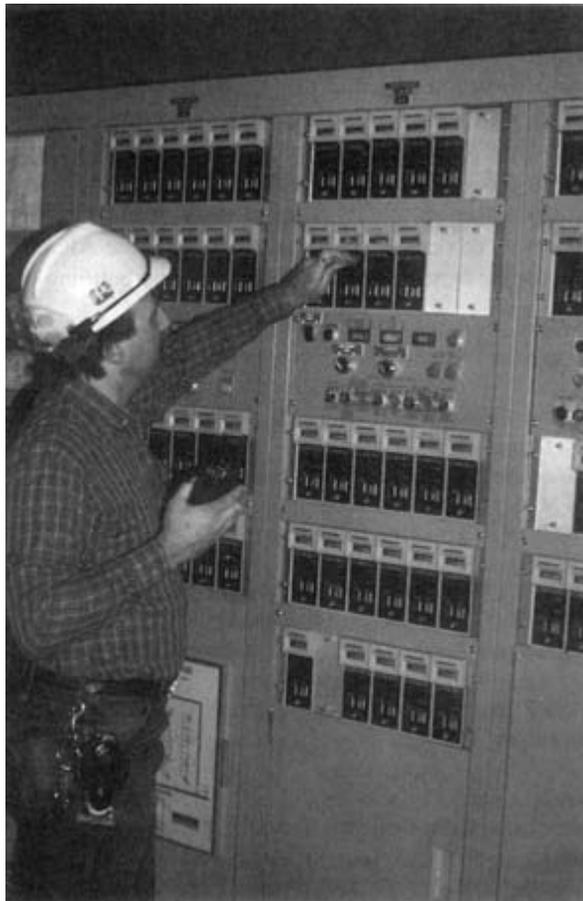
FIGURE 10-25 An instrument mechanic proof-tests a critical instrument panel.
