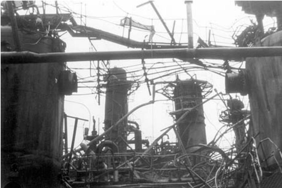
FIGURE 5-16 A Destroyed Section of the Flixborough Reactor System.
