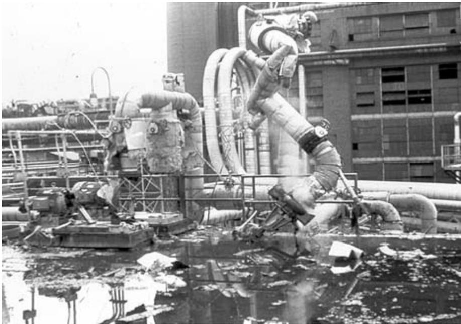
FIGURE 7-15 Heavily damaged condensate pump installation. Courtesy of Eastman Chemical Company.
