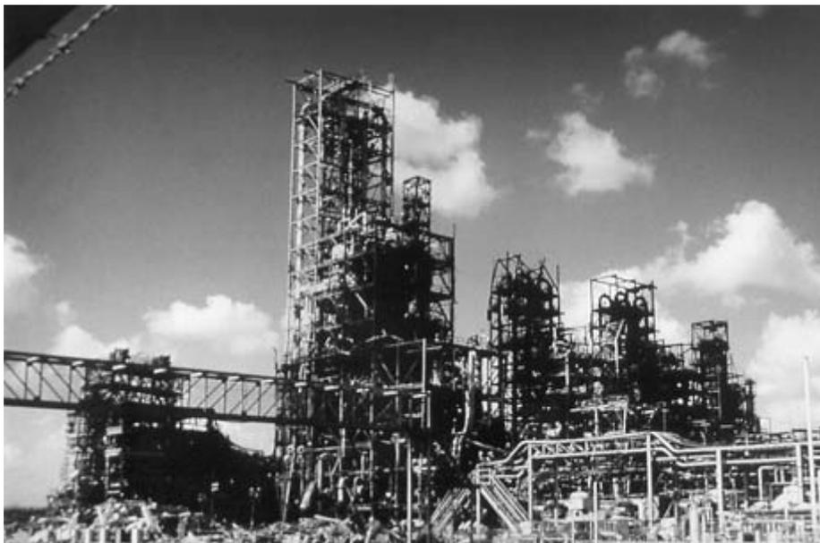
FIGURE 5-6 A ground-level view of the charred structure and destruction at Phillips 66.
