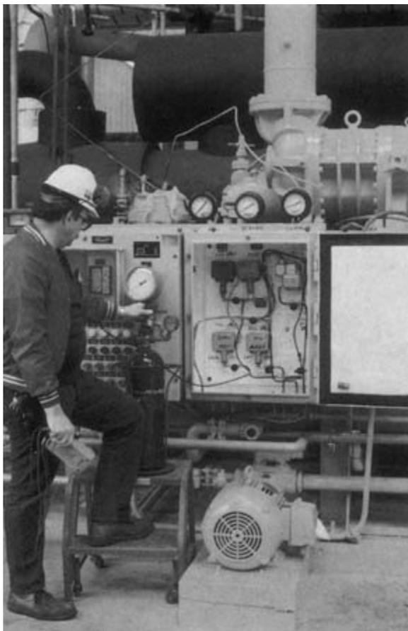
FIGURE 10–22 Prooftesting a high-pressure switch on a refrigeration unit.
