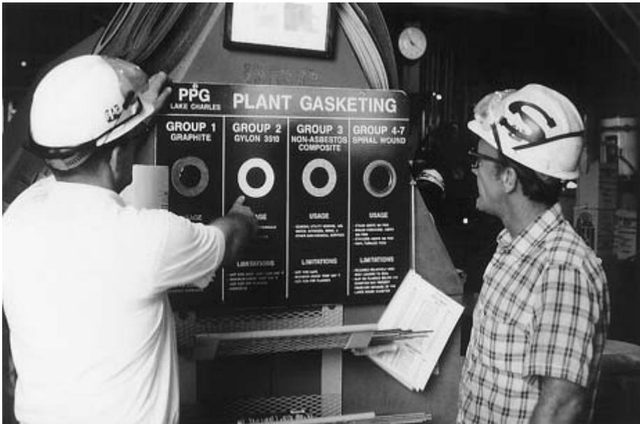
FIGURE 6-9 Choosing the proper piping gaskets with help from easy-to-understand gasket board.
