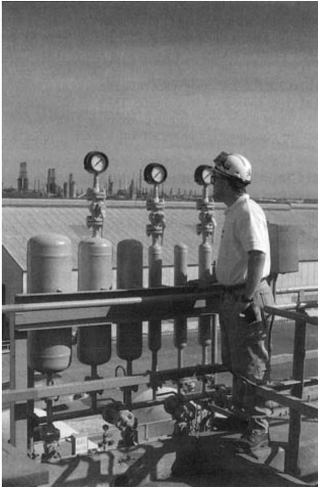
FIGURE 4-5 An engineer observes the pressure gauges on chlorine expansion bottles.
