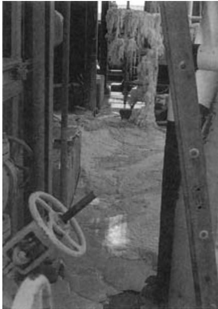
FIGURE 6-6 Molten caustic soda leaks from above due to an improper gasket.
