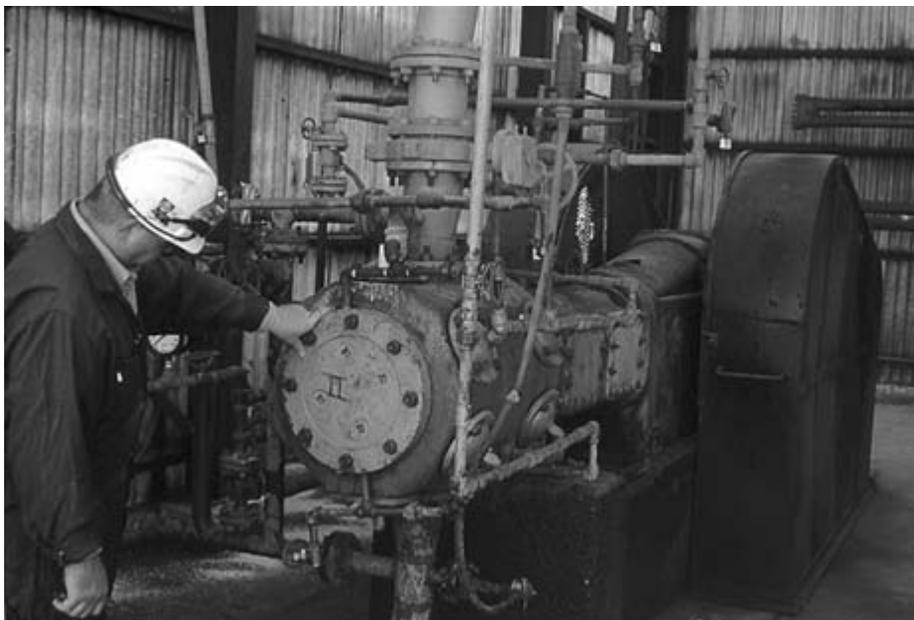
FIGURE 7-3 Rebuilt reciprocating compressor.
