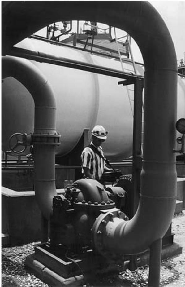
FIGURE 10-2 A vibration technician taking readings on a cooling water pump.
