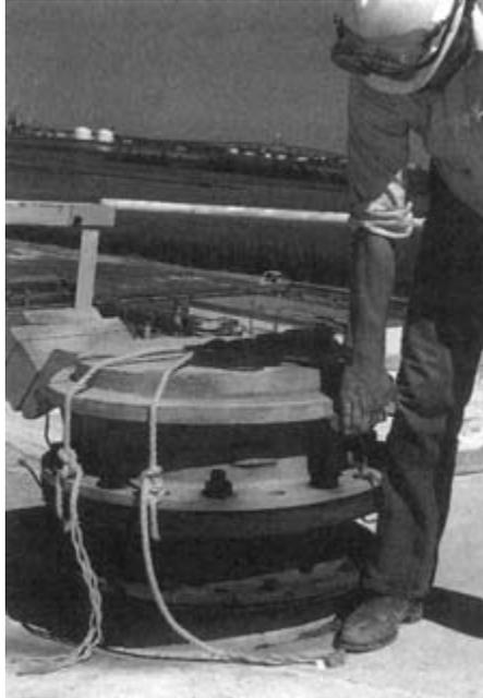
FIGURE 6–10 Hinged vent lid improperly tied to cope with anticipated high winds and to prevent intrusion of rain.
