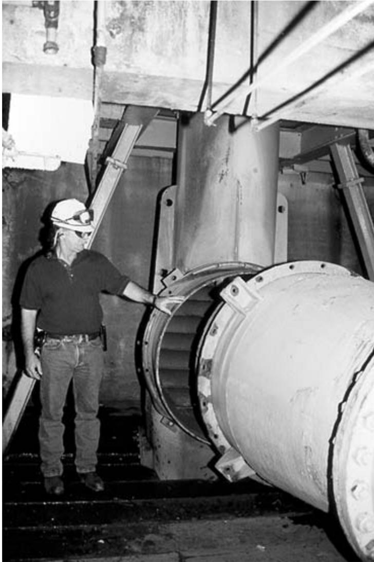
FIGURE 7-9 Photo of how the river water pump moved during the explosion.
