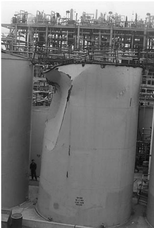
FIGURE 2-16 Crushed tank in the tank farm.
