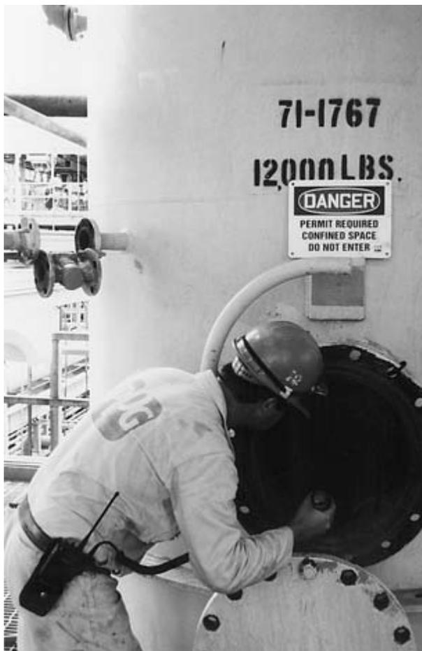
FIGURE 10-9 A pressure vessel inspector making an initial assessment of the vessel and determines any special inspection needs, such as ladders, scaffolding, or extra lighting.
