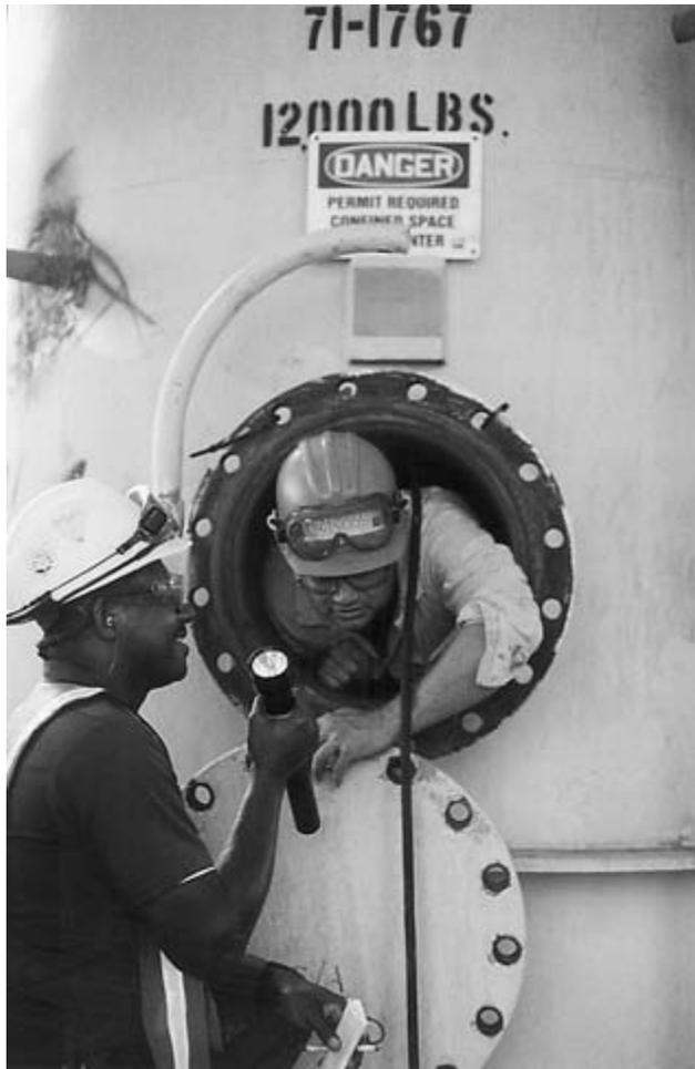
FIGURE 10–10 A pressure vessel inspector enters the confined space after the vessel is blinded, tested, and cleared, but still relies on a manway watch.
