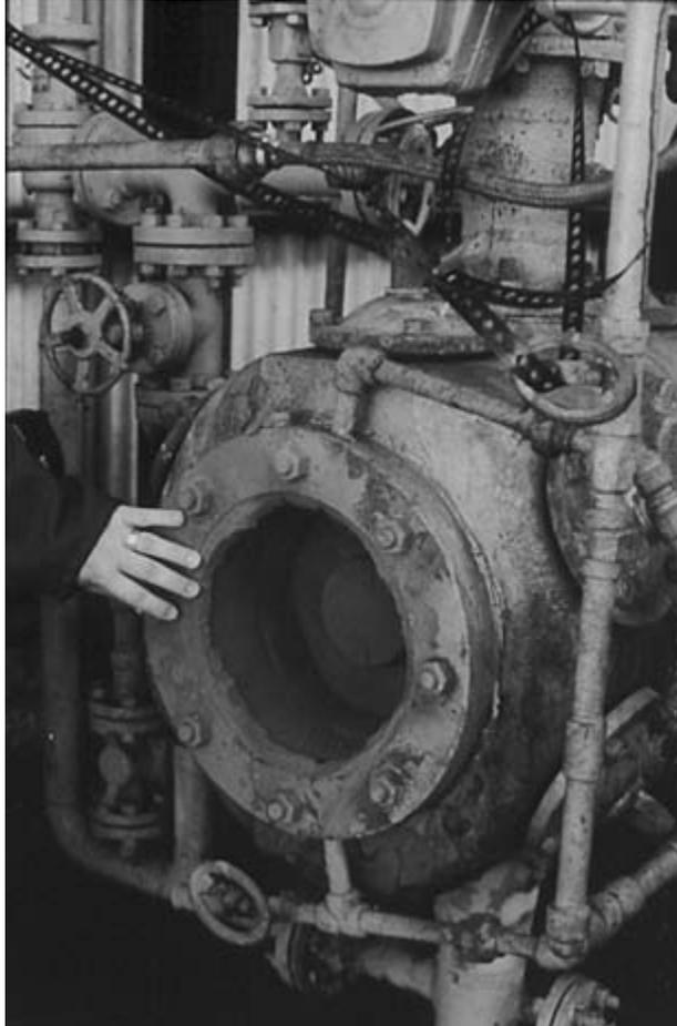
FIGURE 7-2 Close-up of ruptured water jacket on compressor.
