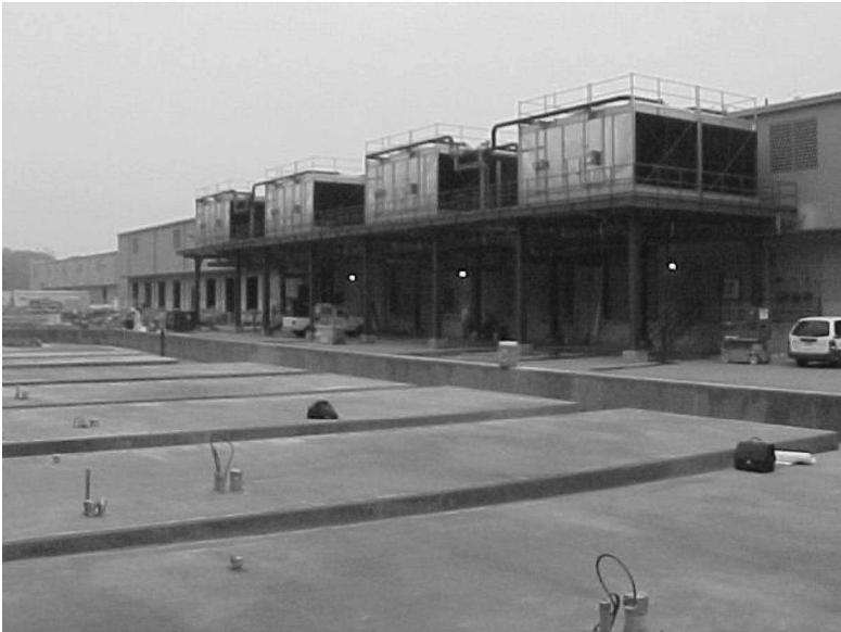
**Figure 11.11** Direct cooling towers on an elevated platform. (Photo courtesy of DLB Associates.)
