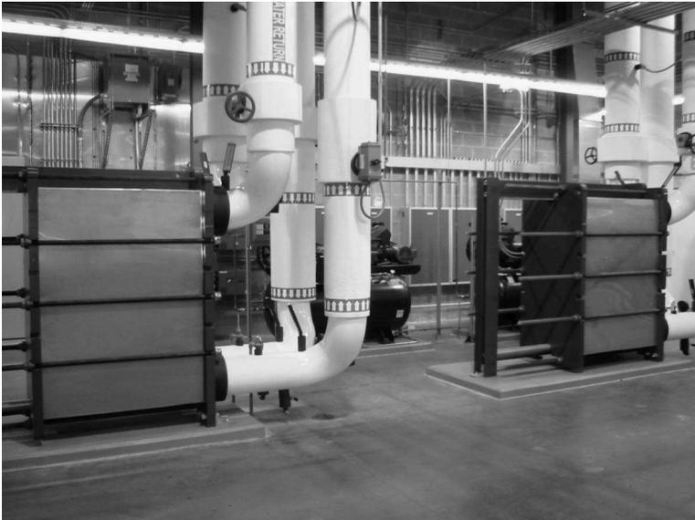
**Figure 11.23** Installed plate and frame heat exchangers. (Photo courtesy of DLB Associates.)
