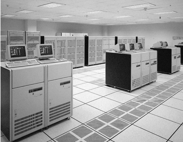
**Figure 12.1** Typical raised floor. (Courtesy of Tate Access Floors.)
