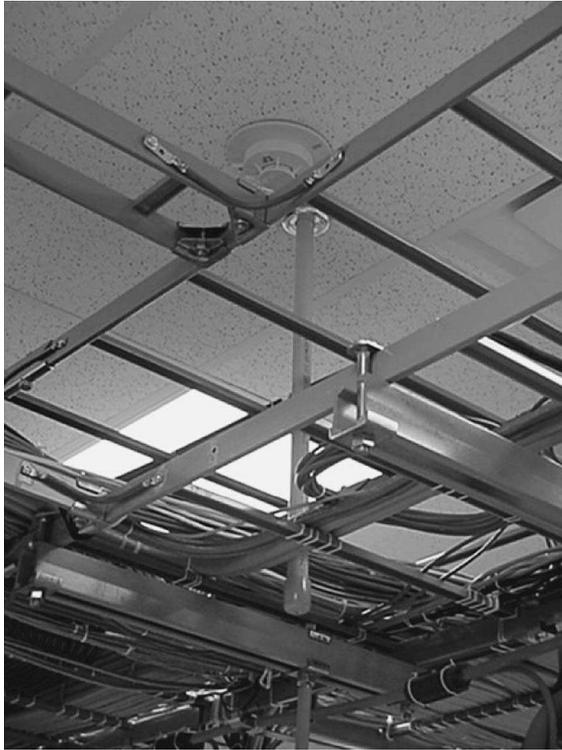
**Figure 13.3** High–low layouts of smoke detectors include some detectors 3 ft below the ceiling to overcome stratification. A spot detector (high) and air-sampling port (low) shown here. (Courtesy Orr Protection Systems, Inc.)
