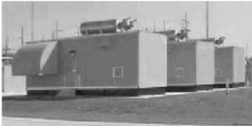
Figure 24 Substation diesel gensets. Source: Cummins Power Generation.
