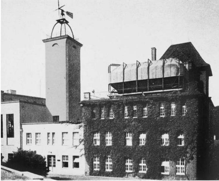
Fig. 9.1 The institute for aerodynamics of the Technical University Aachen with its new Göttingen-type wind tunnel on the roof [546].
