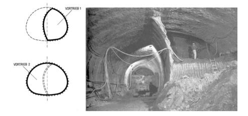
Fig. 9. Experiment – Compressed-air tunnel driving in the shotcrete construction method, 1979 Line5/9 Munich Odeonsplatz [1]
