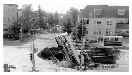
Fig. 1. Munich Trudering collapse, Subway line 2 - East Section 2 [9]
