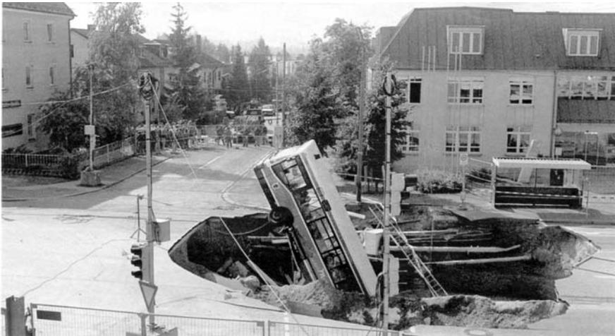
**Fig. 1.** Munich Trudering collapse, Subway line 2 - East Section 2 [9]
