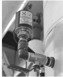
The diaphragms are typically made from stainless steel which allows them to be used with water and other corrosive fluids. In some applications, **silicon diaphragm** sensors are available that are useful for high frequency measurements. These devices have their strain gauges bonded to them by atomic diffusion during manufacture.
