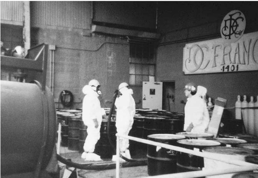
**Figure 9-3.** Pump-out of paint drums for off-site disposal.
