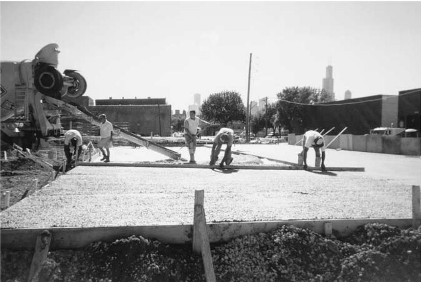
**Figure 9-11.** A reinforced concrete cap was installed.
