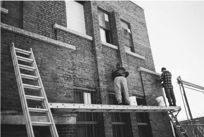
**Figure 9-5.** Repairing and tuckpointing brickwork.
