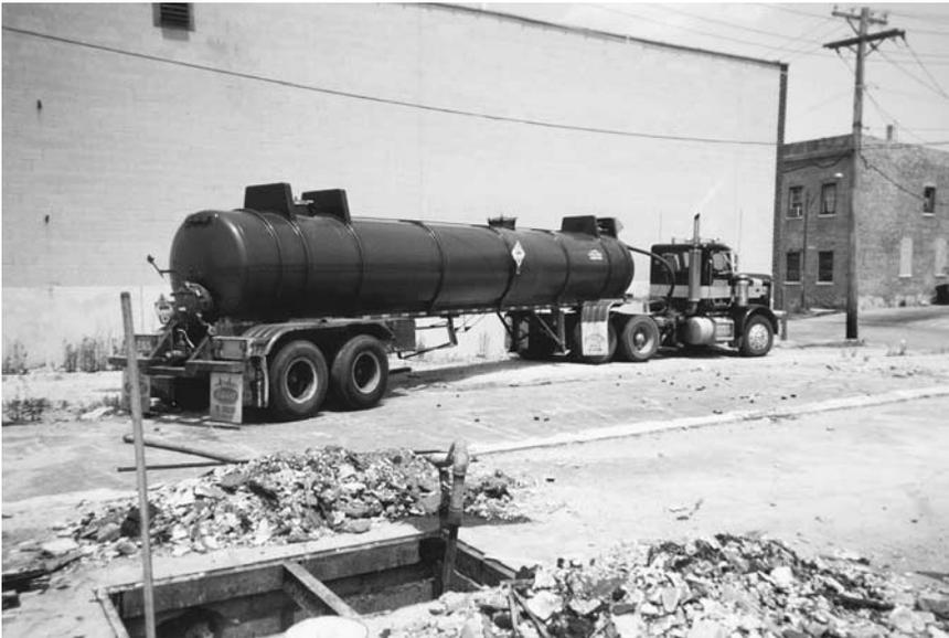
**Figure 9-9.** Two 20,000-gallon underground fuel oil tanks were pumped out.
