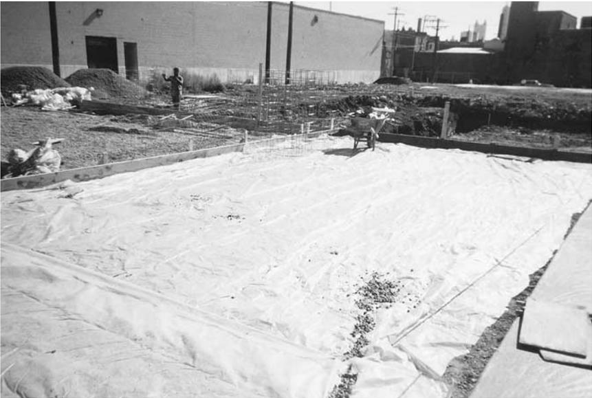
**Figure 9-10.** A vapor barrier was installed as part of an engineered barrier.
