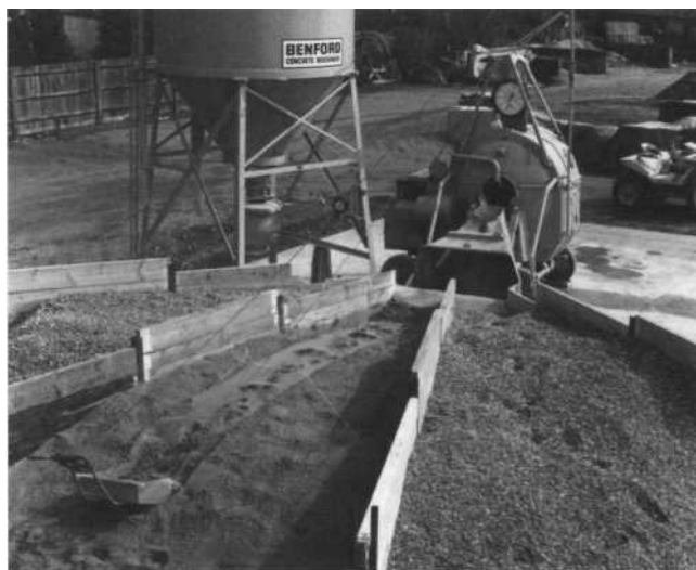
Figure 14: Typical site batching and mixer set-up with drag-line skip for loading the hopper.
