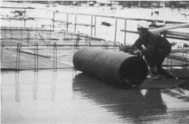
Figure 23: Laying a thermal blanket on a freshly finished slab.
