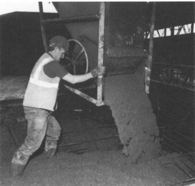
Figure 16: Roll-over skip with wheel-controlled discharge mechanism.
