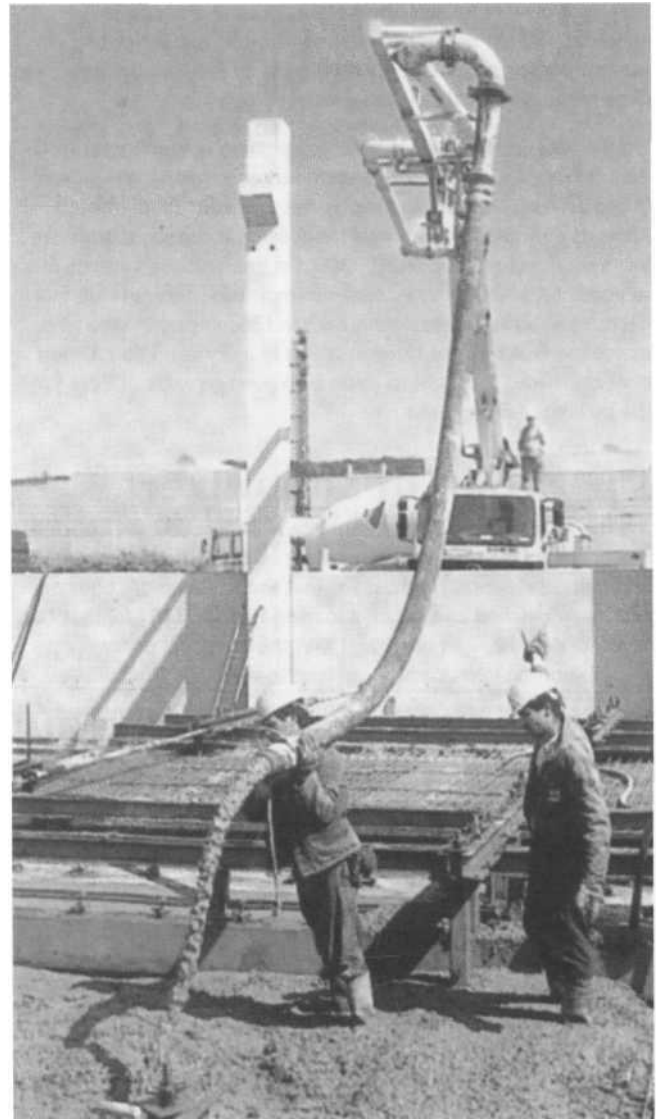
Figure 15: Placing by pump.
