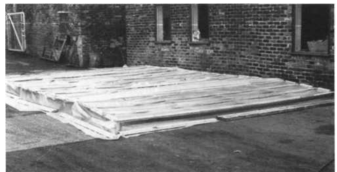
Figure 11: Polythene sheeting supported clear of a concrete slab by means of blocks and timber. Note that all the edges of the polythene are held down to prevent a wind-tunnel effect.
