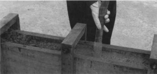
Figure 19: The concrete is fully compacted in the immediate vicinity of the poker
