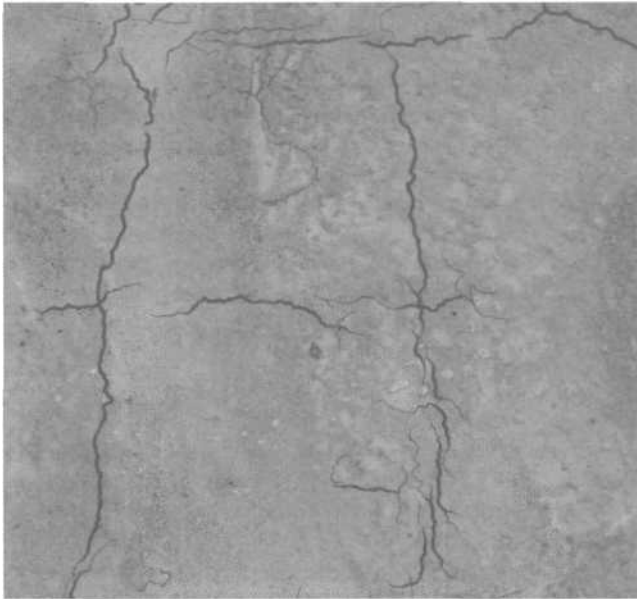
Figure 8: Plastic settlement cracks mirror the reinforcement.
