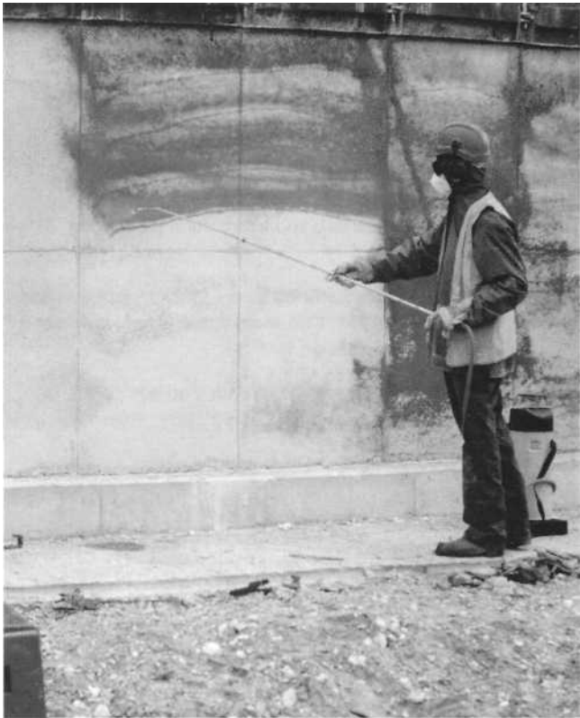
Figure 30: Spraying a reservoir wall with a curing membrane.
