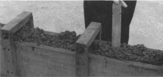
Figure 18: Inserting a poker in fresh (stiff) concrete in a beam.
