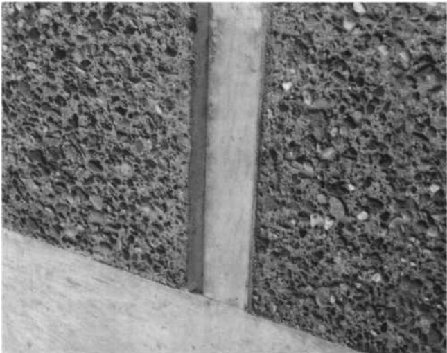
Figure 31: An example of an in-situ exposed-aggregate finish obtained with the aid of a surface retarder.
