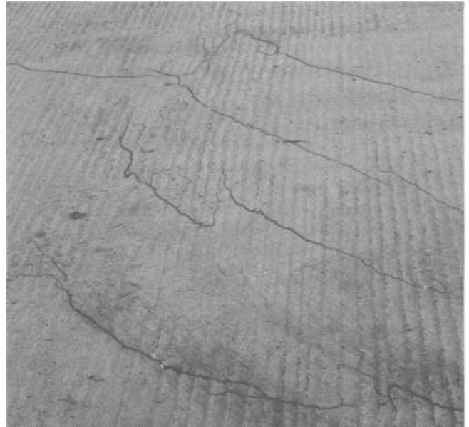
Figure 10: Plastic shrinkage cracks in a concrete road
