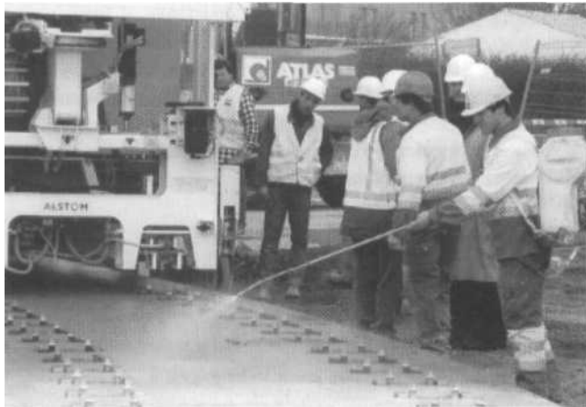
Figure 24: Applying a sprayed-on curing membrane to freshly laid concrete.
