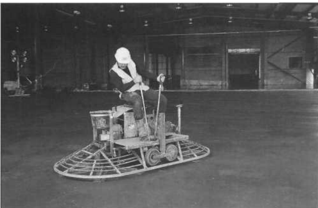
Figure 33: Power trowelling an industrial floor slab.
