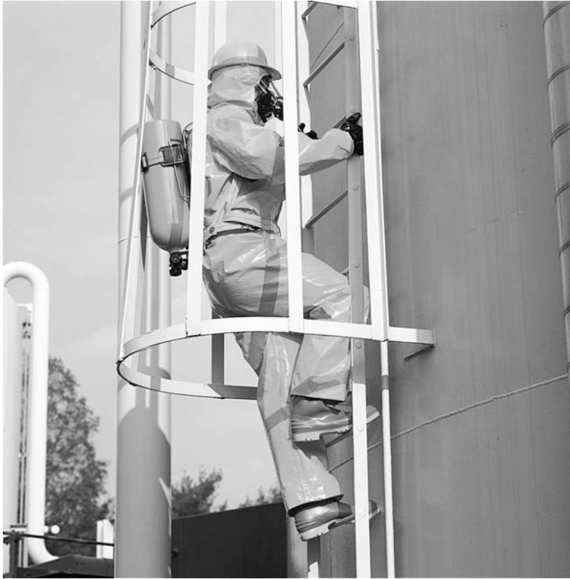
FIGURE 9-5. This worker appears to be ascending a caged ladder. Note the likelihood of airlines or apparatus becoming entangled in the cage when the worker is on the descent. Photo courtesy of DuPont Tyvek®/ Tychem® protective apparel
