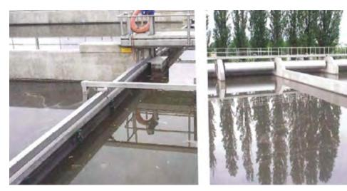
**Figure 8.8** process stages at the Markranstadt wastewater treatment. Left: inflow chamber to the membrane bioreactor with overflow edge to combined water treatment, right: combined water treatment tank.
