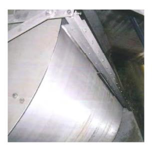
Figure 8.3 Rotary screen of the fine screen installation
