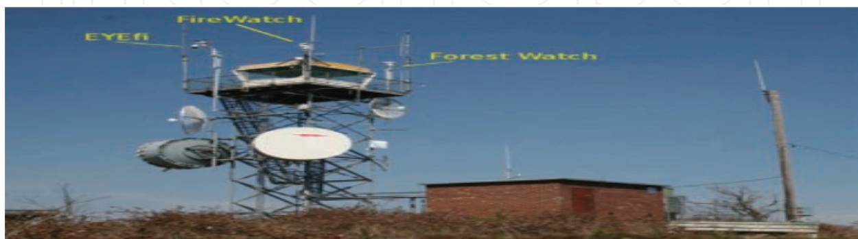
Figure 11. Tower in Tumut, Australia, with the three systems [20].
