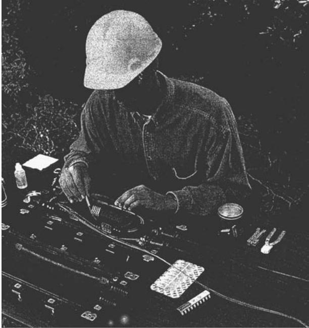
**FIGURE 4.9** Craftsman populating an aerial closure with mechanical splices. (Fiber cleaver at right, bottle of index-matching gel at left.) [3M]
