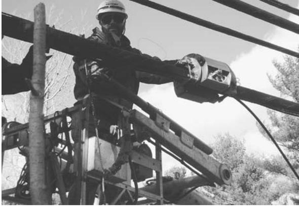
**FIGURE 4.4** Typical installation of lashed aerial fiber cable.
