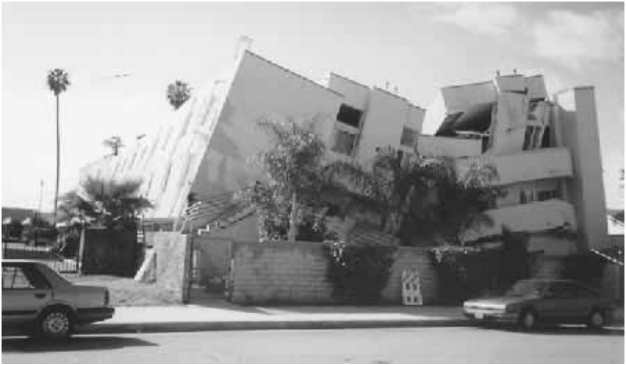
FIGURE 4.6 Building collapse caused by a soft story due to the parking garage on the first floor. The building collapse occurred during the Northridge earthquake in California on January 17, 1994.
