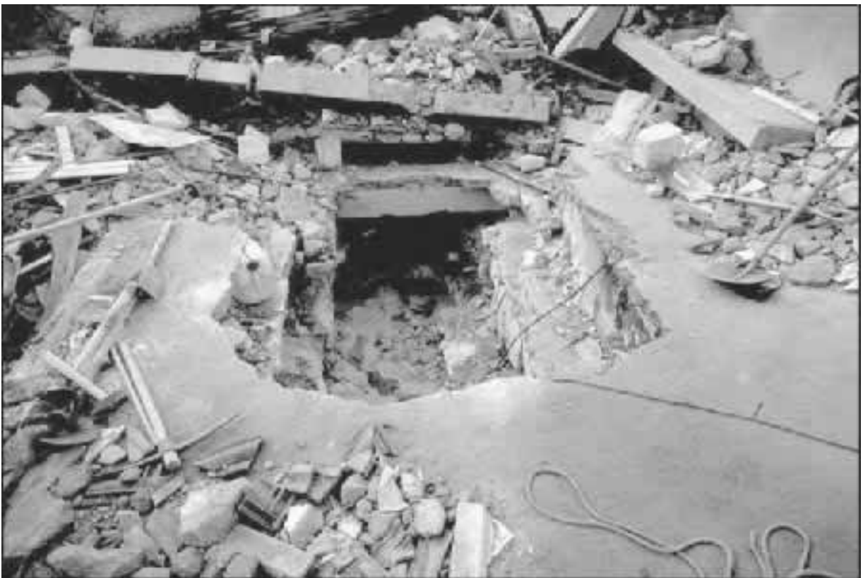
FIGURE 4.16 Pancaking of a building, during the Izmit earthquake in Turkey on August 17, 1999. Note that the center of the photograph shows a hole that was excavated through the pancaked building in order to rescue the survivors. (Photograph from the Izmit Collection, EERC, University of California, Berkeley.)
