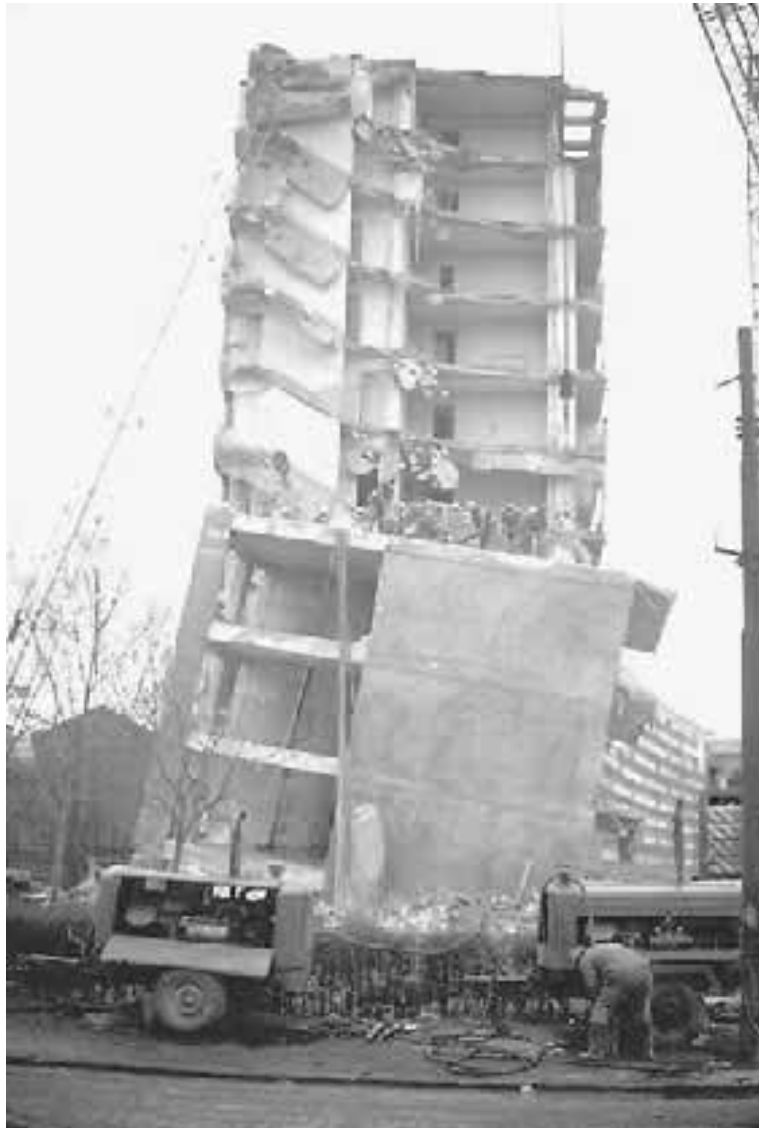
FIGURE 4.19 A comparatively new building that was proclaimed as “earthquake-proof” because of the box-type construction consisting of numerous shear walls. Nevertheless, the structure was severely damaged because of earthquake-induced settlement of the building during the Bucharest earthquake on March 4, 1977. (Photograph from the Steinbrugge Collection, EERC, University of California, Berkeley.)
