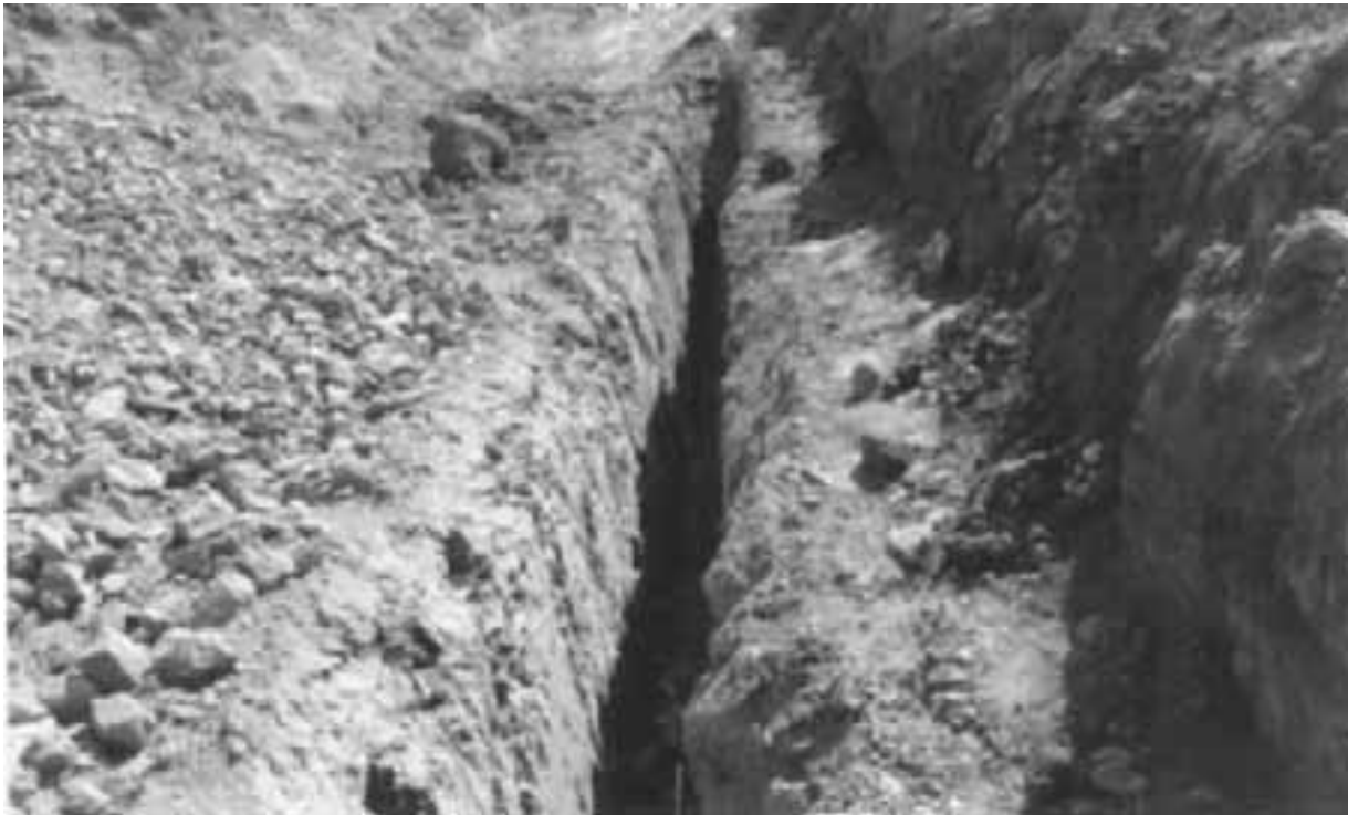
FIGURE 5.8 Backhoe trench for a fault study.
