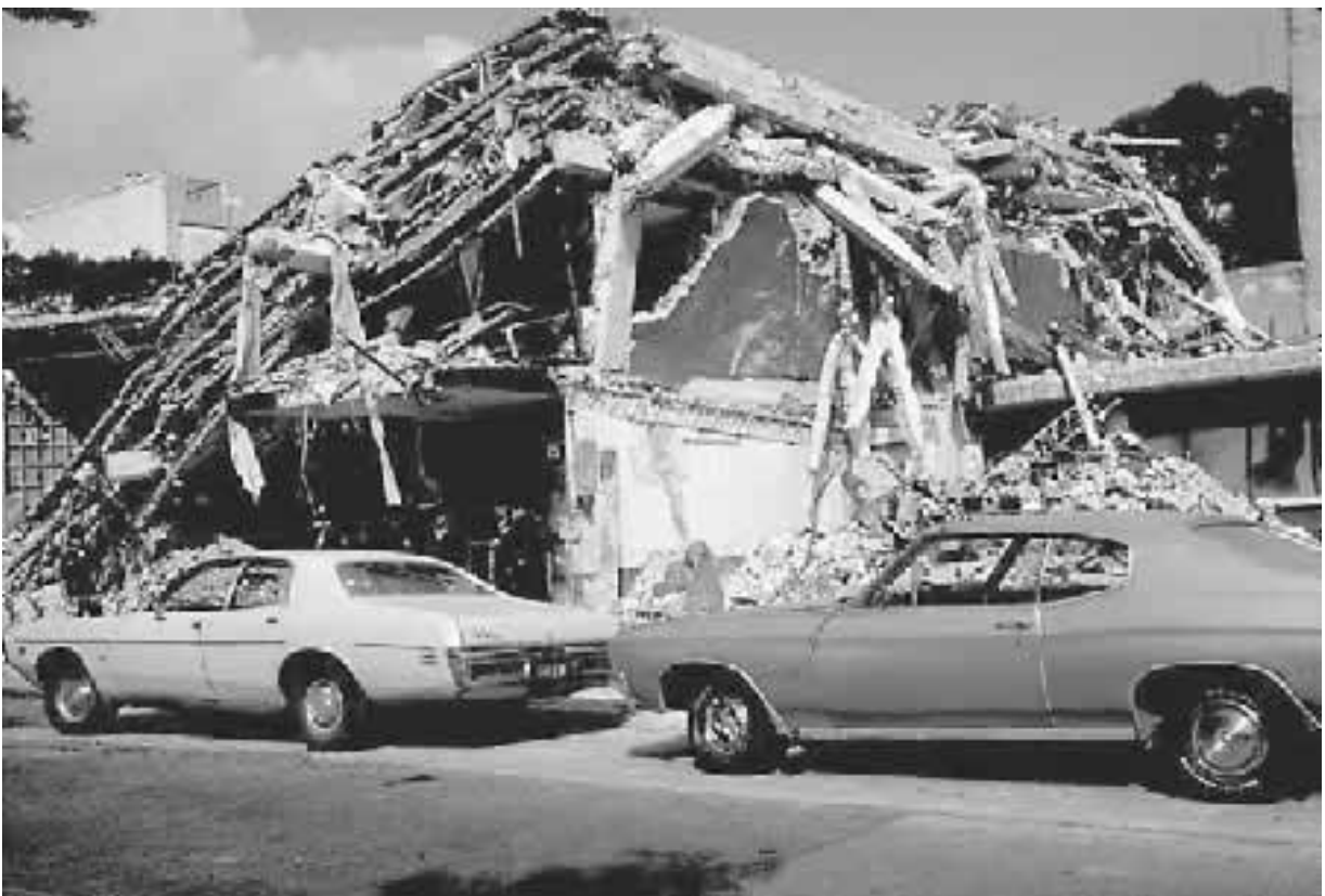
FIGURE 4.24 Building collapse in Mexico City caused by the Michoacan earthquake in Mexico on September 19, 1985. (Photograph from the Steinbrugge Collection, EERC, University of California, Berkeley.)
