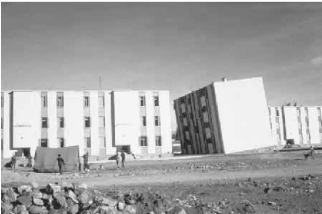
FIGURE 4.11 Building tilting and damage caused by a soft story due to a ground-floor crawl space. The damage occurred during the El Asnam earthquake in Algeria on October 10, 1980. (Photograph from the Godden Collection, EERC, University of California, Berkeley.)
