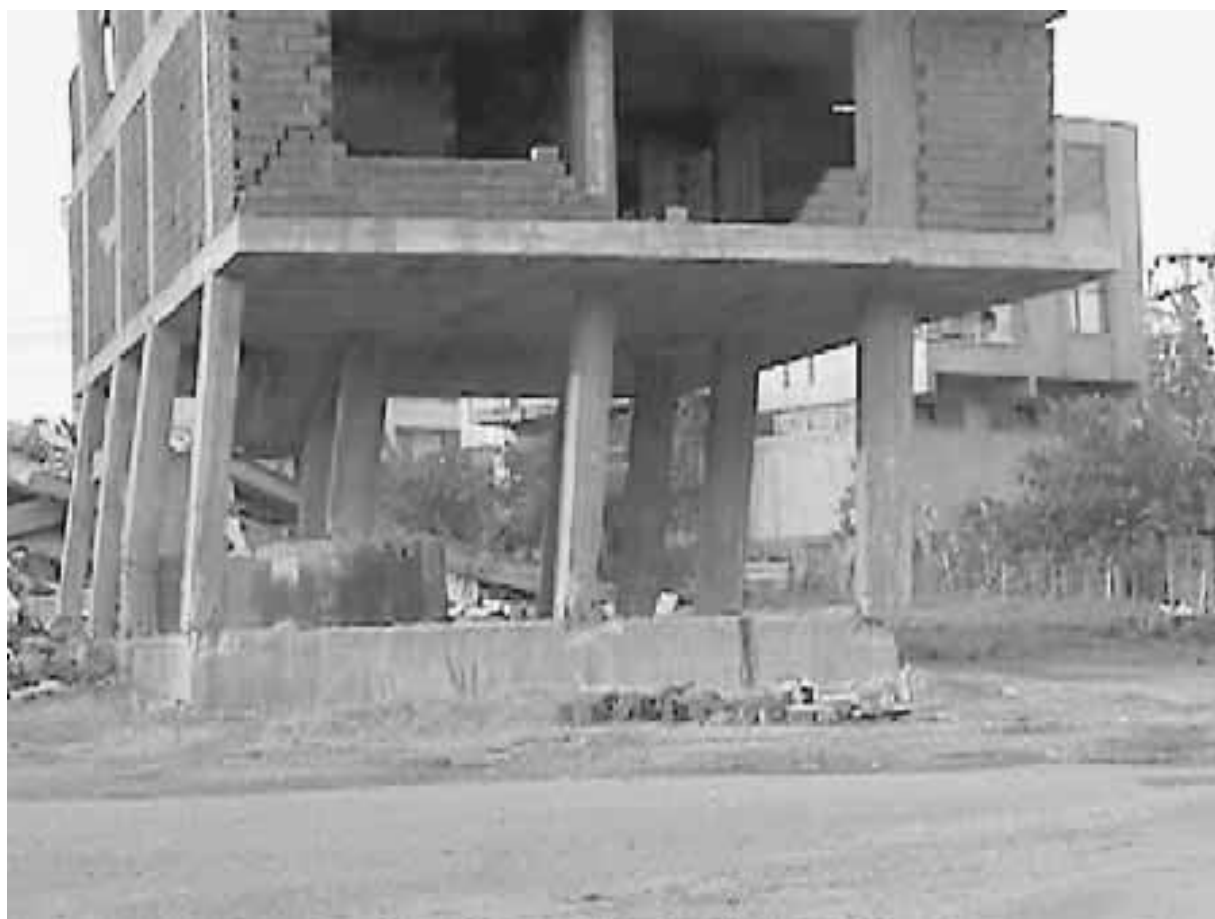
FIGURE 4.9 Damage caused by a soft story at the first-floor level. The damage occurred during the Izmit earthquake in Turkey on August 17, 1999. (Photograph by Mehmet Celebi, USGS.)
