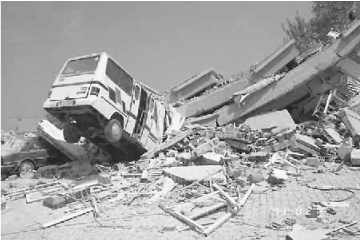
FIGURE 4.15 Pancaking of a building, which also partially crushed a bus, during the Izmit earthquake in Turkey on August 17, 1999. (Photograph from the Izmit Collection, EERC, University of California, Berkeley.)
