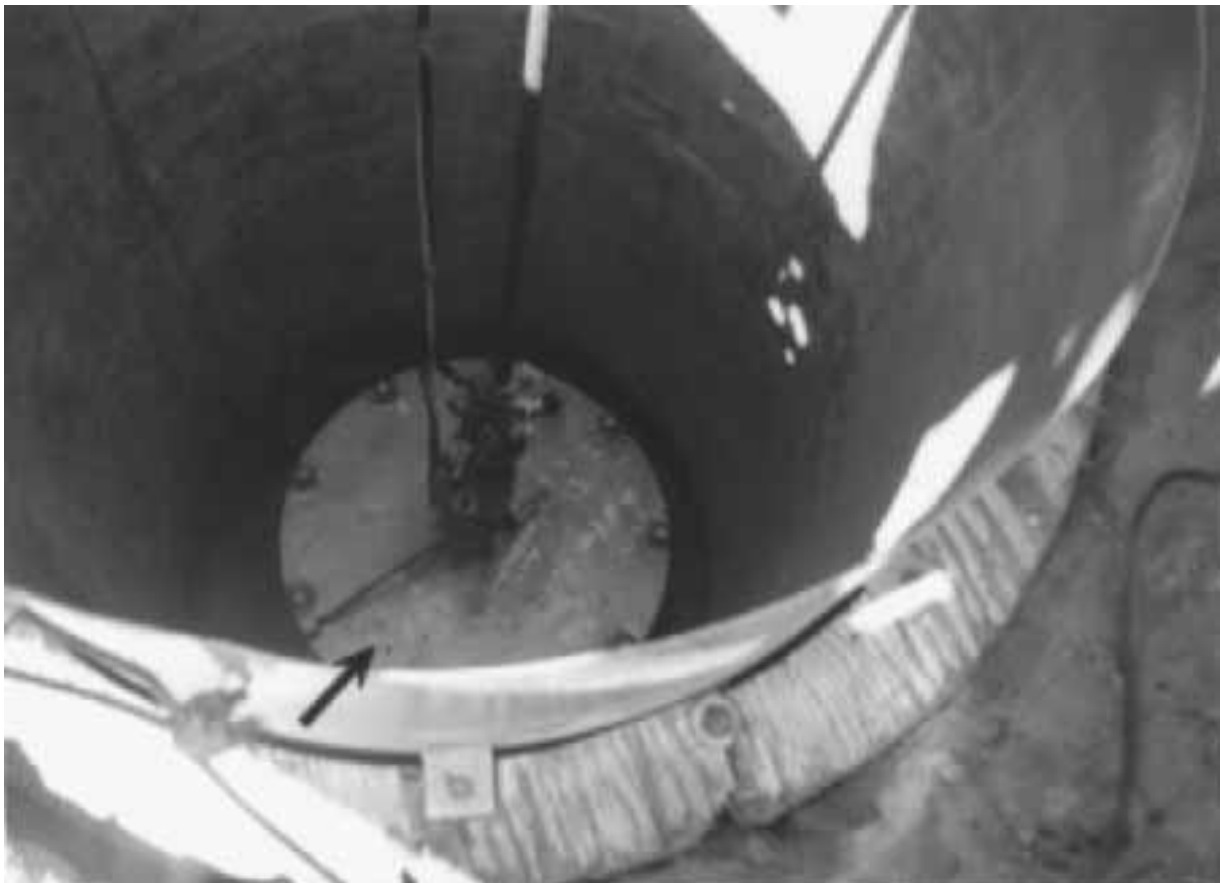
FIGURE 5.5 Down-hole logging. Note that the arrow points to the top of the steel cage used for the down-hole logging.
