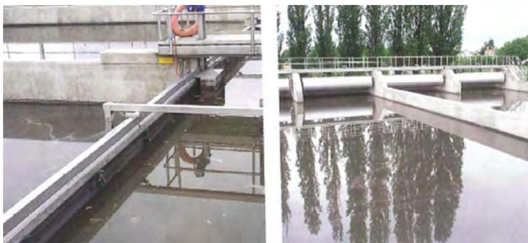
**Figure 8.8** process stages at the Markranstadt wastewater treatment. Left: inflow chamber to the membrane bioreactor with overflow edge to combined water treatment, right: combined water treatment tank.
